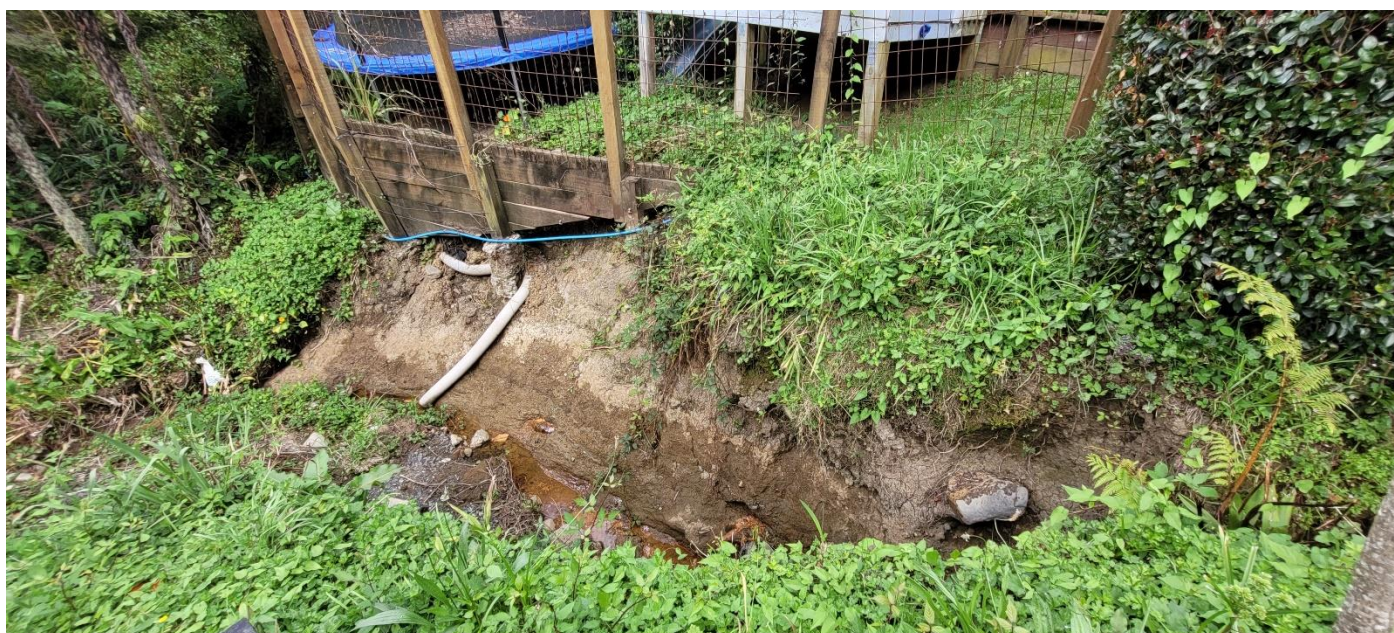
Photo 2: Northern elevation of RTW-02, looking southeast.
