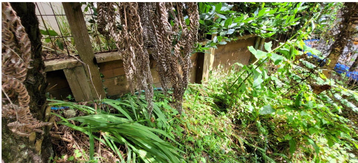
Photo 6: Looking southwest towards the east end of RTW-01.
