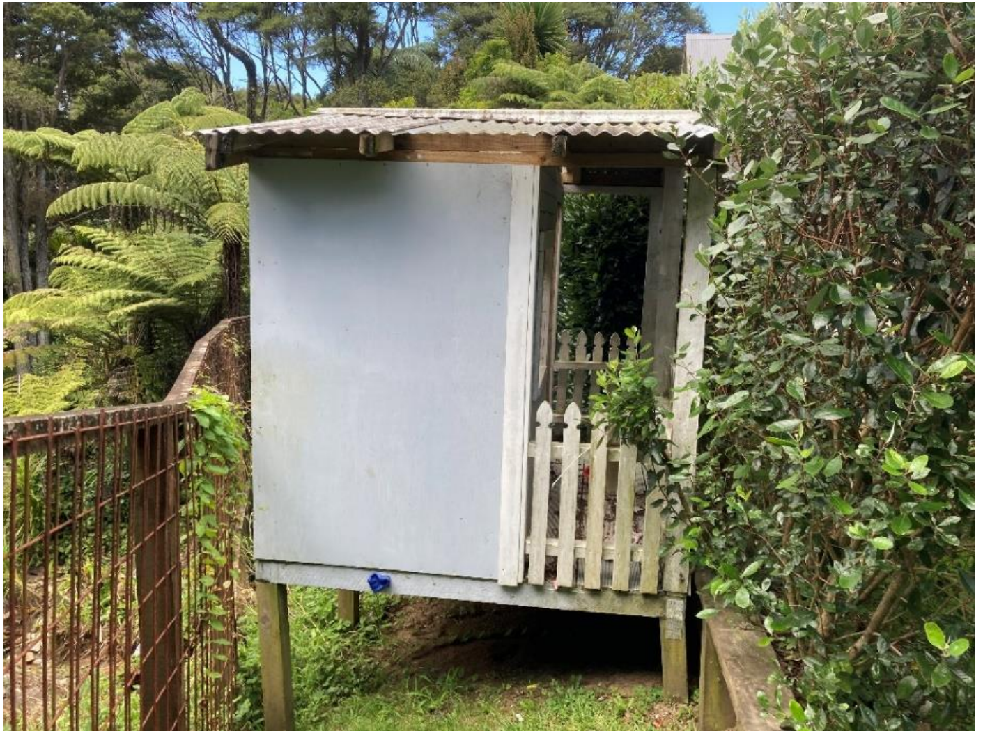
Photo 7: Western elevation of the playhouse, looking east.
