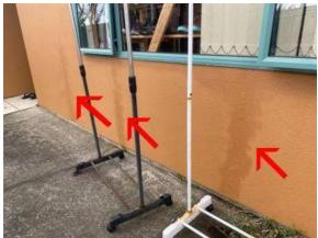
Paved ground level in close proximity to cladding base. A clearance of 100mm is recommended from cladding base to paved ground level to allow adequate cladding drainage. We recommend modifying paving height to meet minimum recommendations and reduce the risk of damage to cladding. Unable to confirm the condition of internal framing in this area at the time of inspection.
