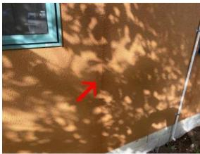
Conduit penetrates exterior cladding. This is considered a high risk detail. Where possible we recommend avoiding cladding penetrations. We recommend monitoring this penetration to ensure a weathertight seal is maintained. As conduit appears to penetrate window head, structural members may have been compromised. We recommend, further inspection to ensure Window lintel has not been compromised.
