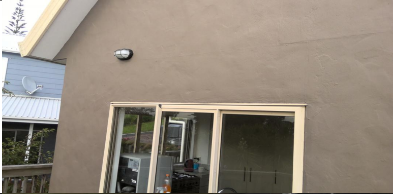
Example of joinery in plaster cladding
