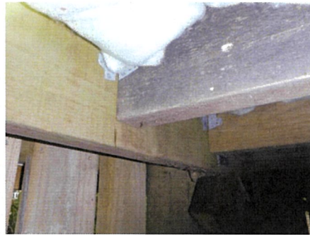
Correct joist hangers recommended
