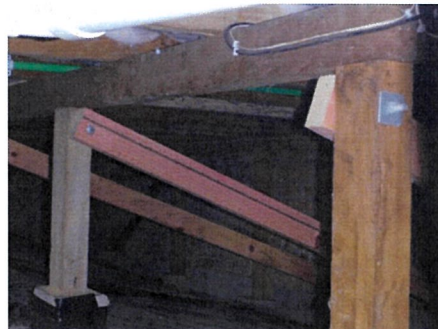
Additional bracing has been installed
