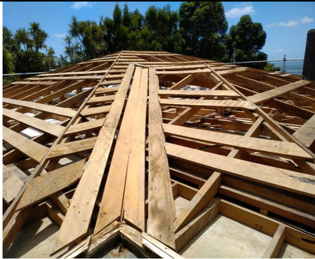
Timber roofing frame work following removal of super 6 roof sheeting.
