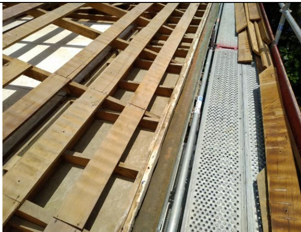
Timber roofing frame work following removal of super 6 roof sheeting.
