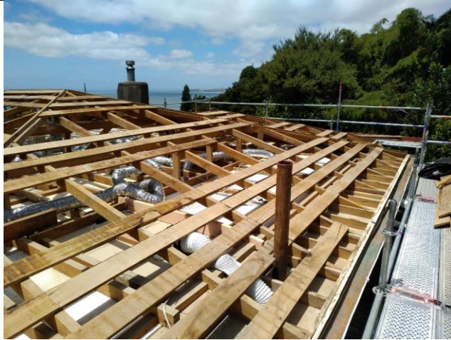
Timber roofing frame work following removal of super 6 roof sheeting.
