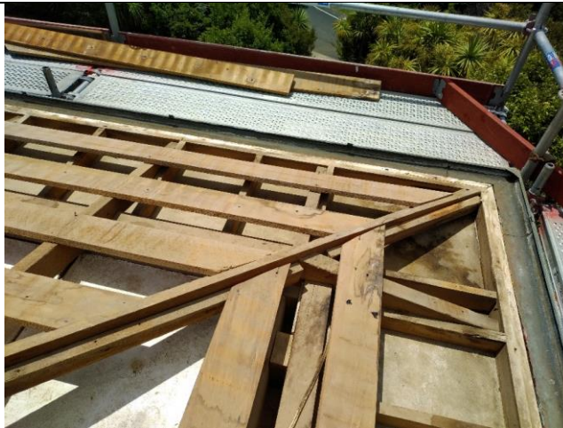
Roof timber frame joints following removal of debris and residues.
