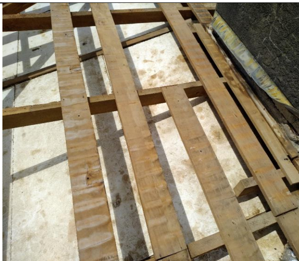
Timber roofing frame work following removal of super 6 roof sheeting.
